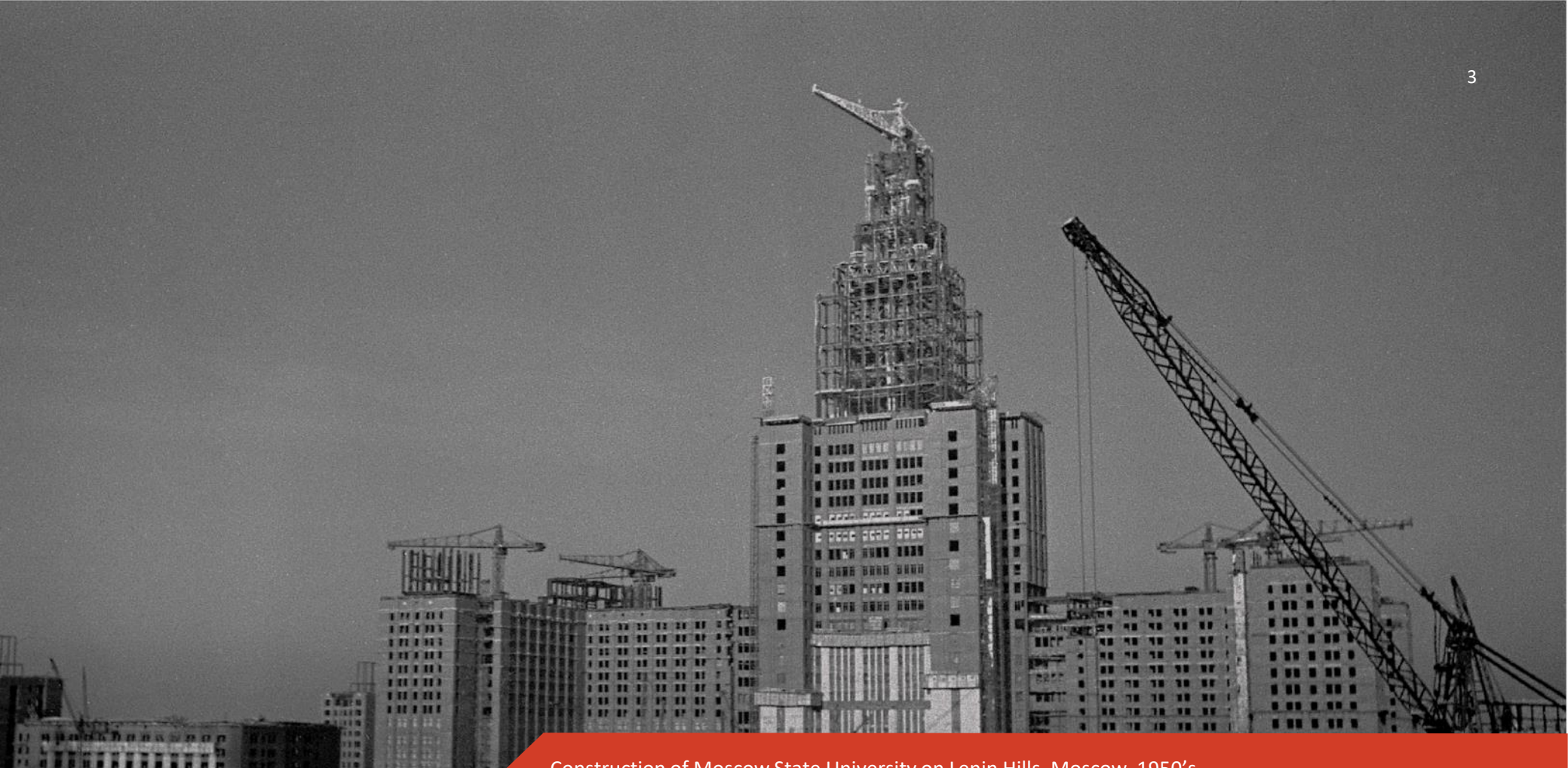
Construction of Moscow State University on Lenin Hills, Moscow, 1950's
